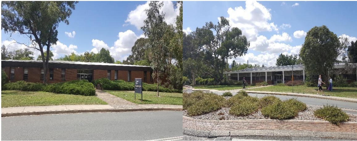
D. A Brown Building (left) and Banks Wing (right)
